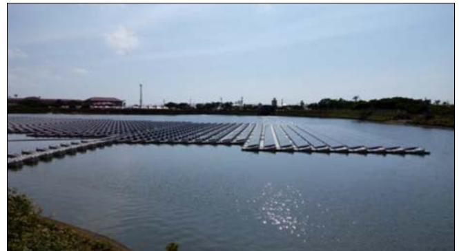
Fig 2: Floating System (FPV).
